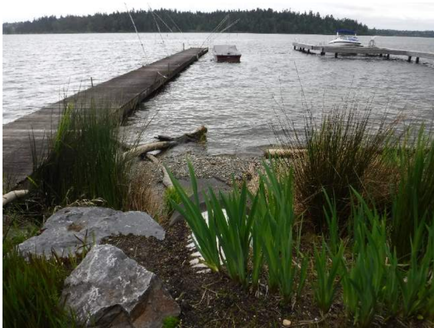
Image 11: Flows outlet the 30" corrugated aluminum pipe and enter Lake Washington
