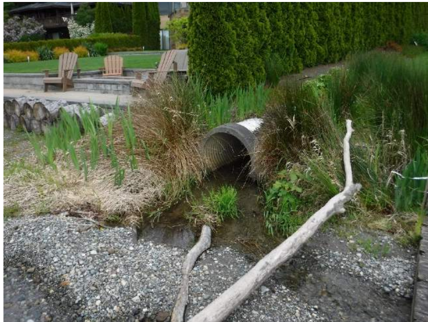
Image 12: Downstream flows outfall into Lake Washington at 5067 SE 51 st St
