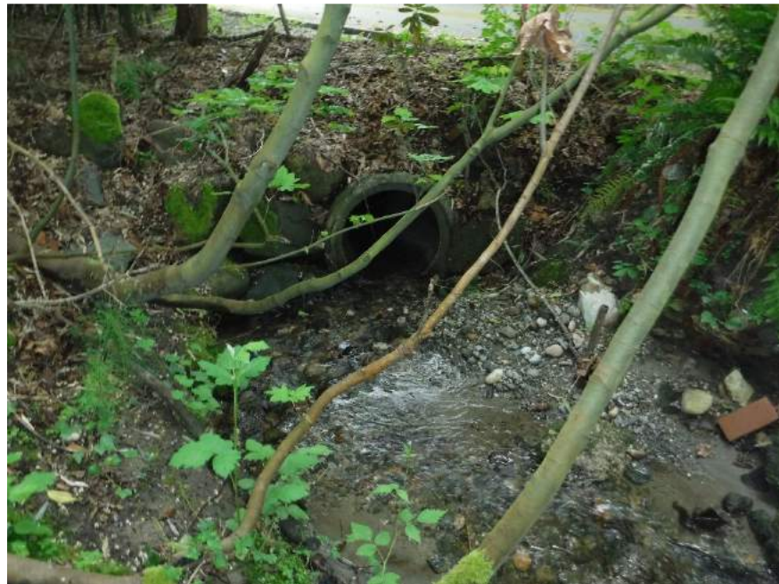
Image 8: Open channel flows inlet this 24" concrete culvert
