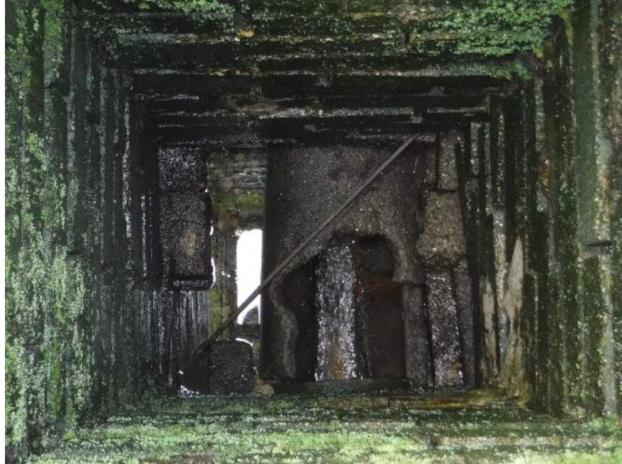
Image 5: Concrete pipe conveys flows through this CB
