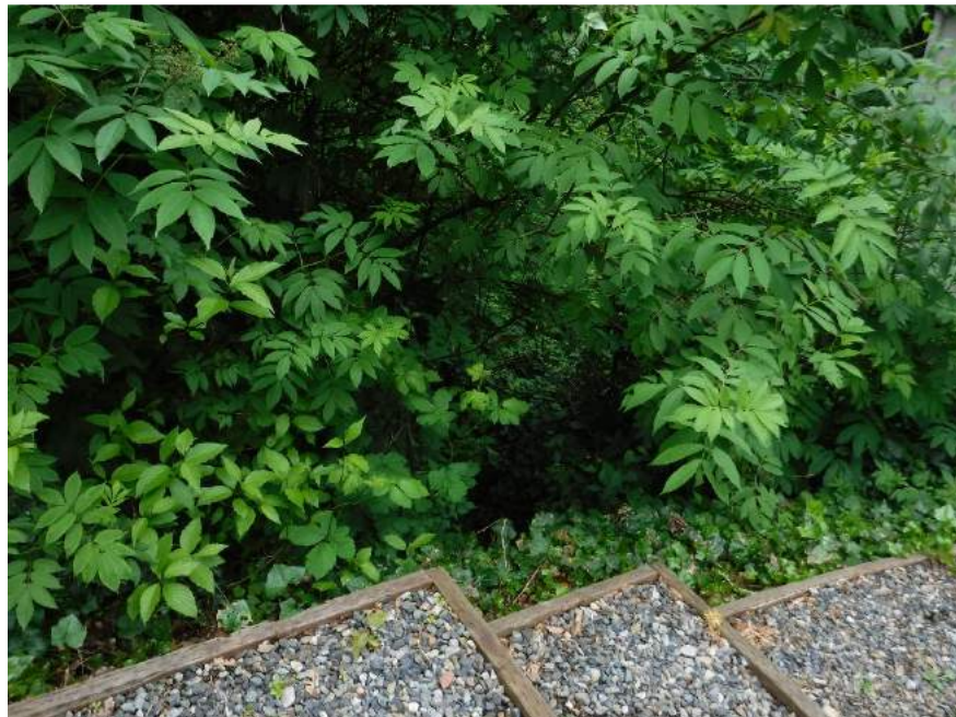
Image 6: Downstream flows outlet to this open channel private watercourse located at 5200 W Mercer Pl
